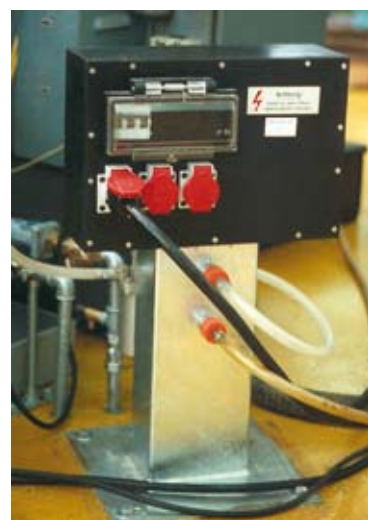
Power distribution for mobile workstation
