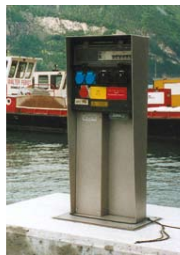
Service/maintenance connections Landing stage
